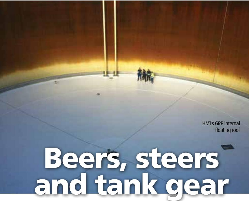
HMT's GRP internal floating roof
